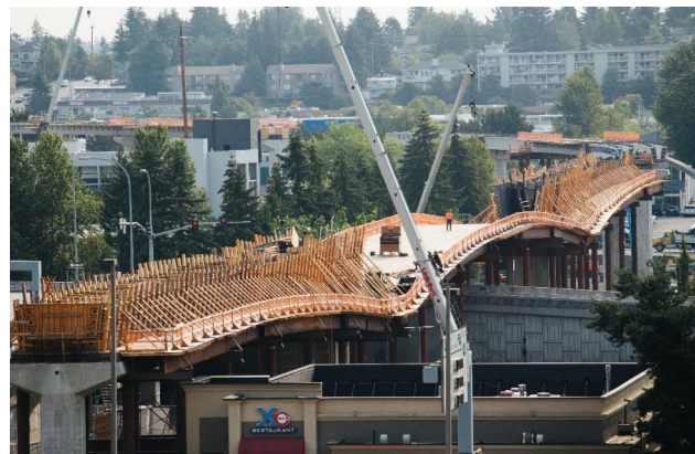
Figure 2-47. Construction of Elevated Guideway Over Roadways
