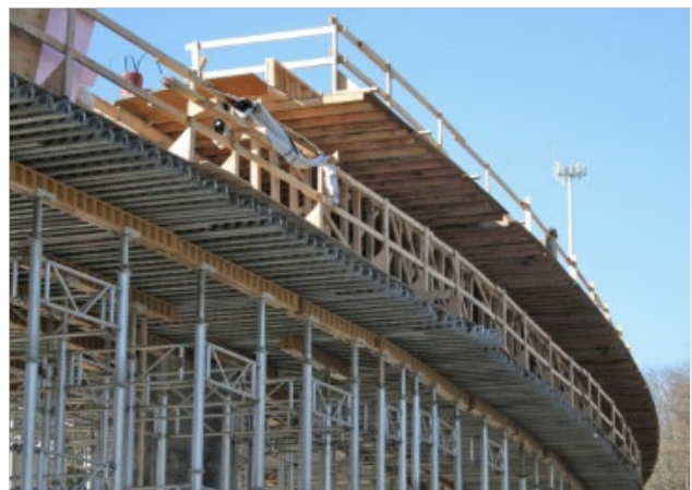
Figure 2-47. Construction of Elevated Guideway Over Roadways
