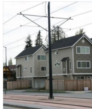
Figure 2-5. Typical Overhead Catenary System
