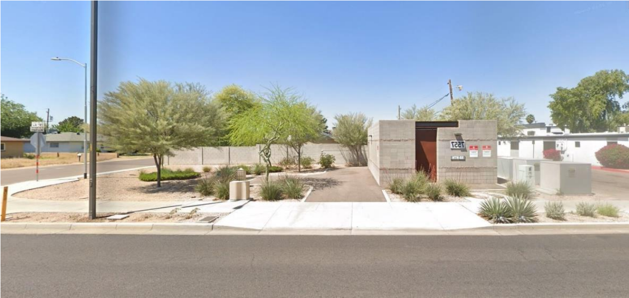
Example Traction Power Substation (Valley Metro, Phoenix, Arizona)
