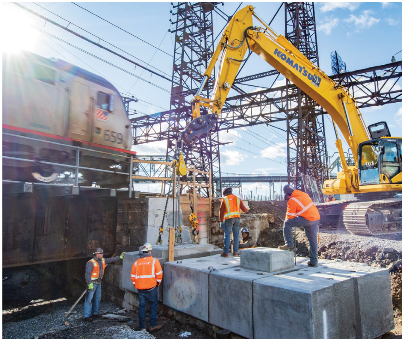
Building a bridge over the Bronx River for the Penn Station Access project
