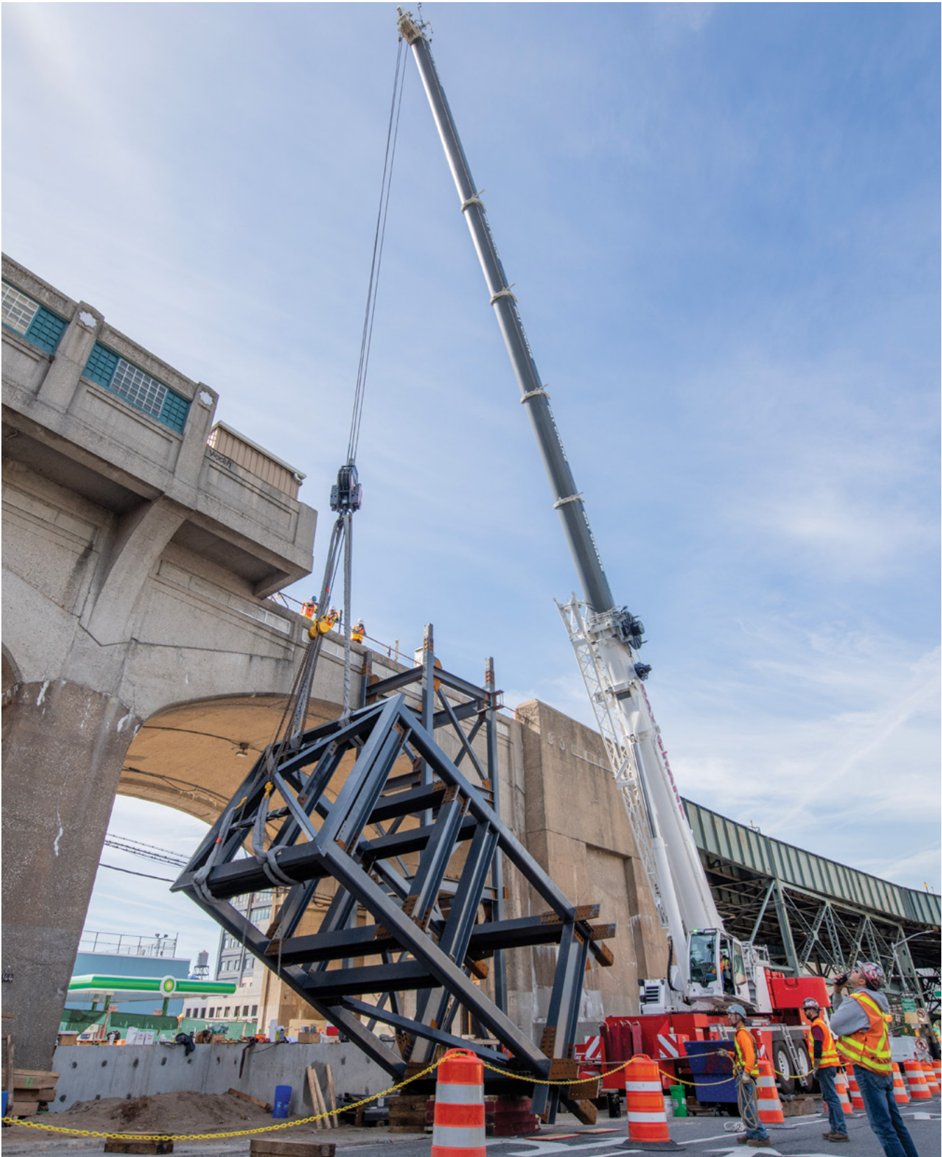
Placing an elevator frame at the 33 St-Rawson St 7 ADA project
