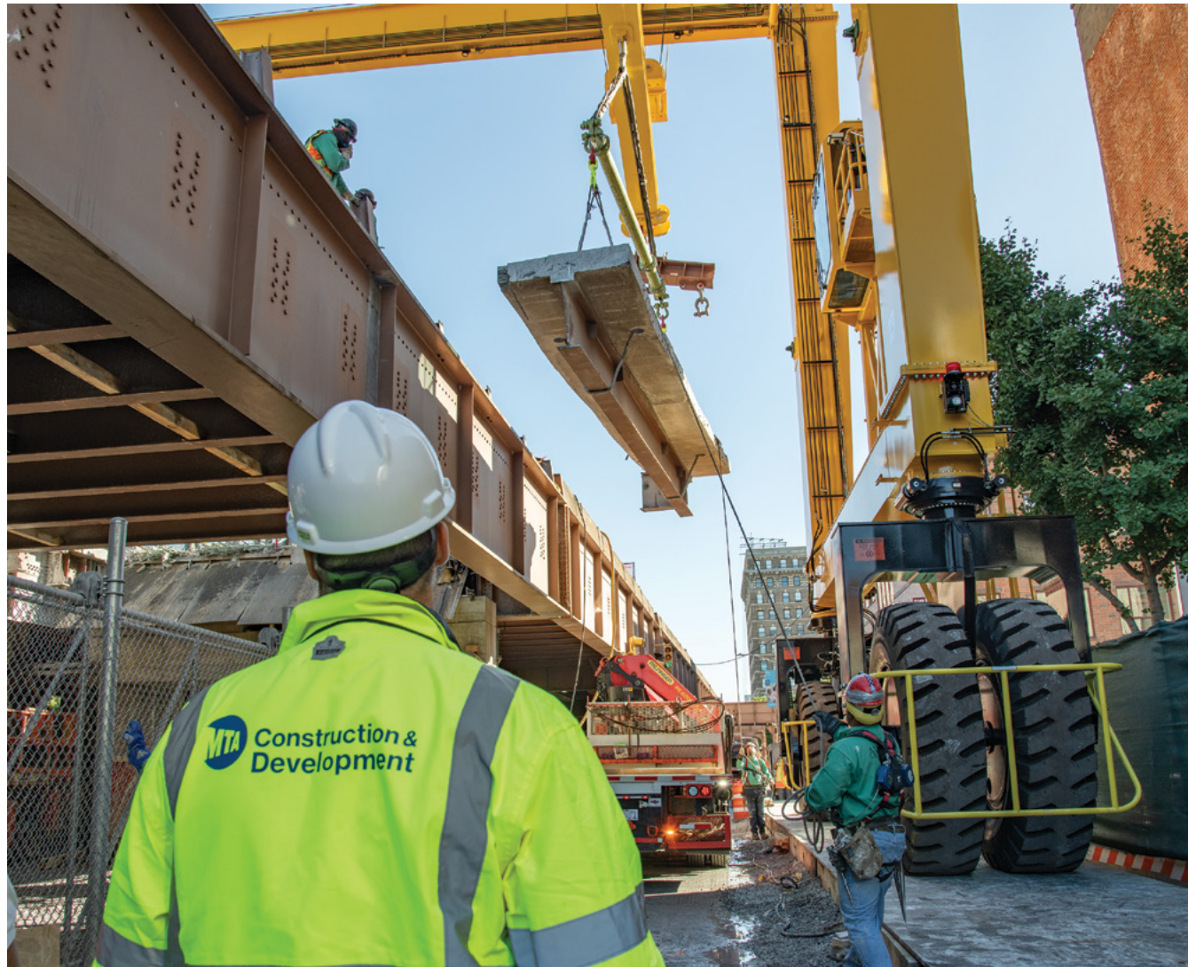
A bridge replacement operation (BRO) on the Park Avenue Viaduct (PAV) project
