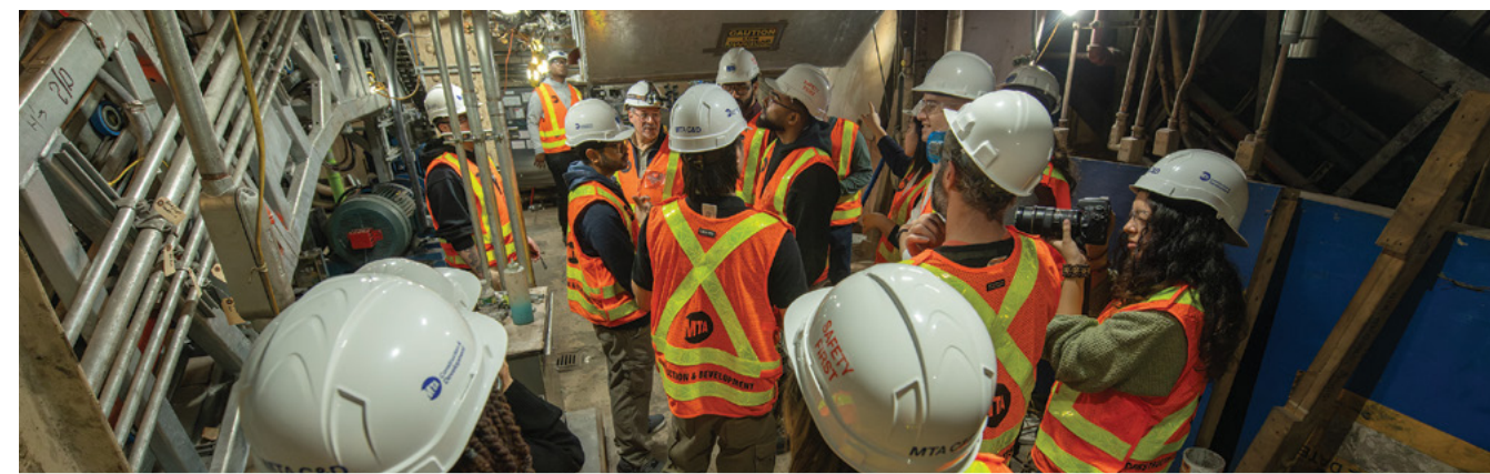
MTA Trainees tour an escalator replacement project
