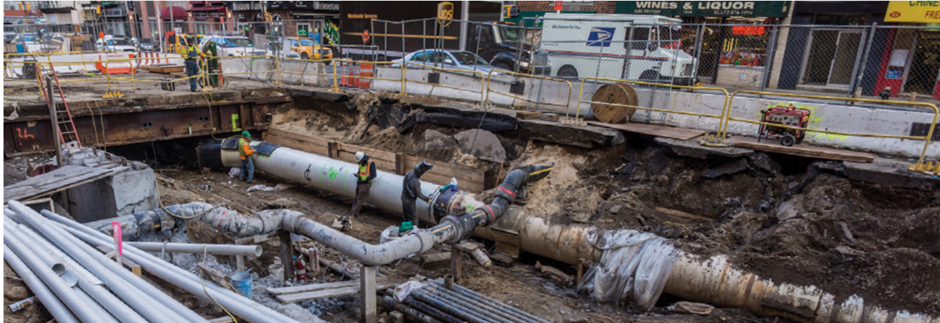
Utility work near 96 St during the Second Avenue Subway Phase 1
